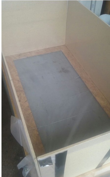
Figure 29: Those would be the side walls from wood to get the part ready for molding. Everything is lined with plastic, but it's hard to see. Basically, a plastic sheet is wrapped around every piece of wood.
