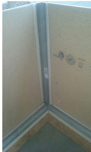
Figure 32: This figure shows the three-way intersection. It will come out of the mold rough, and it will be sanded to a smooth round corner.
